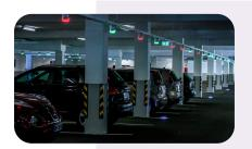
Parking Guidance Cameras detects a vehicle in a space and shows its availability status automatically by colored lights, so drivers can easily see where to park. For example, it turns red for occupied and green for free. Different colors can also be used to categorize spaces, for instance for disabled parking.
