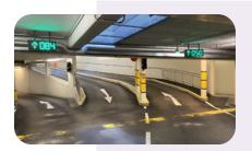
The number of available spaces can be displayed, for example at the entrance to a car park on an LED Display. This uses count information using ANPR data from entrance/exit cameras or Parking Guidance Cameras, and updates immediately when a space fills, or becomes free. It informs a driver right from the start if there's space inside the car park.
