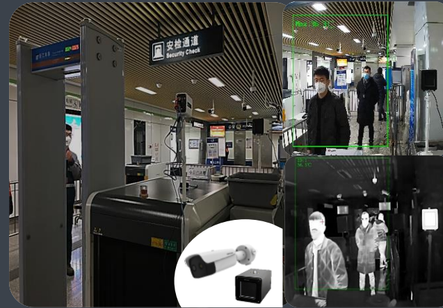
Fixed infrared temperature measurement at entrances of building
