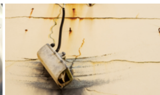
Loosen installation due to corrosion
