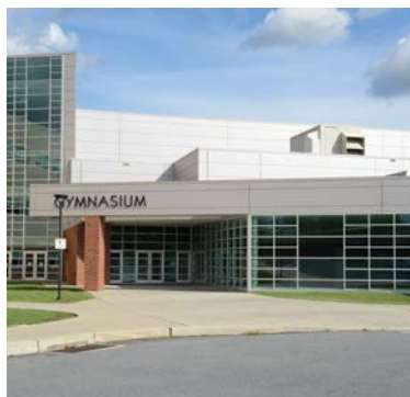
School Entrances & Parking Lots
