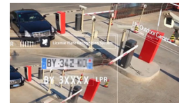
Access control barrier by license plate
