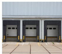
LOADING BAYS & DOCKS
