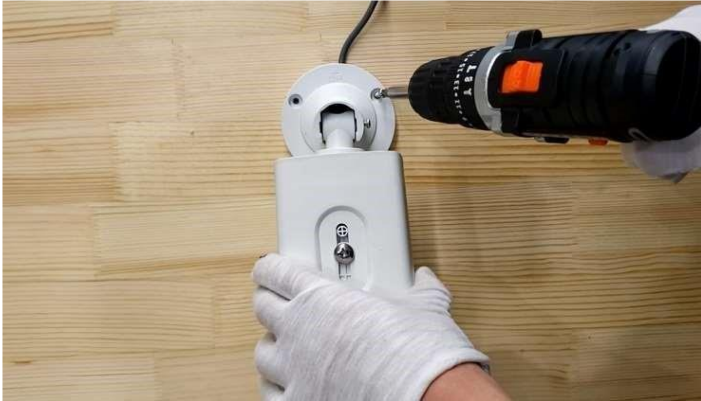
d) Loosen the screws and adjust the lens angel to modify device angel
