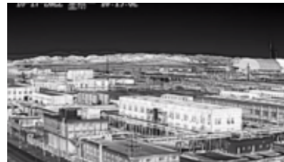
Plant Elevated Position
