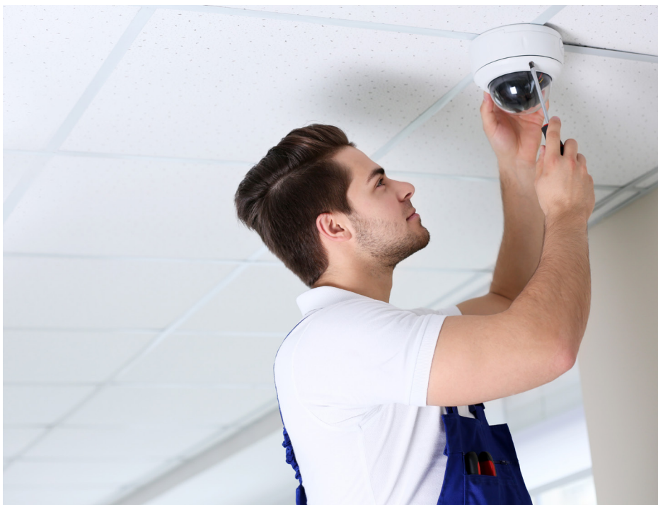
If a camera is to be installed in a patient's room, the room should be enclosed and shut down for a time
