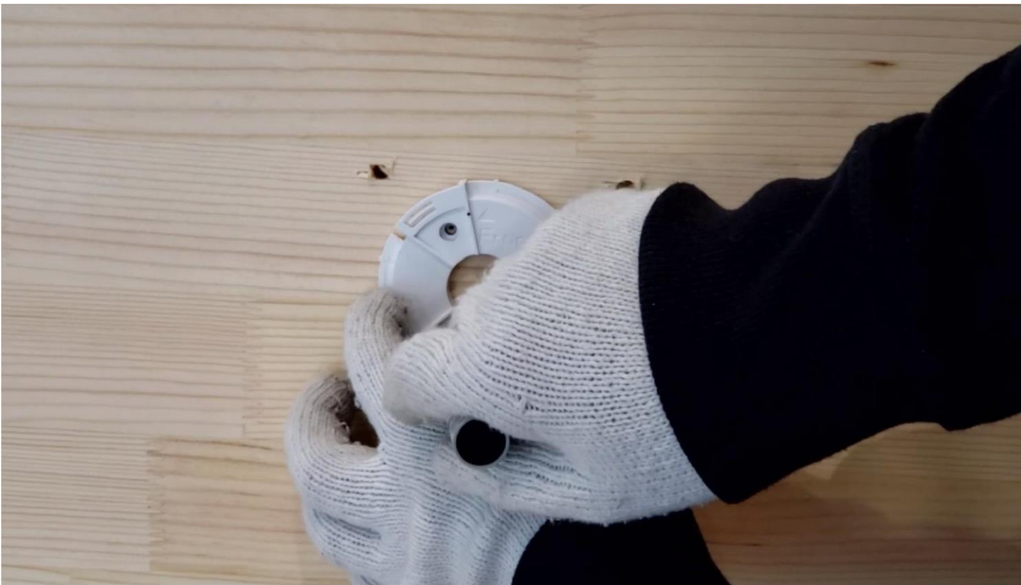
c) Drill holes according to the marks
