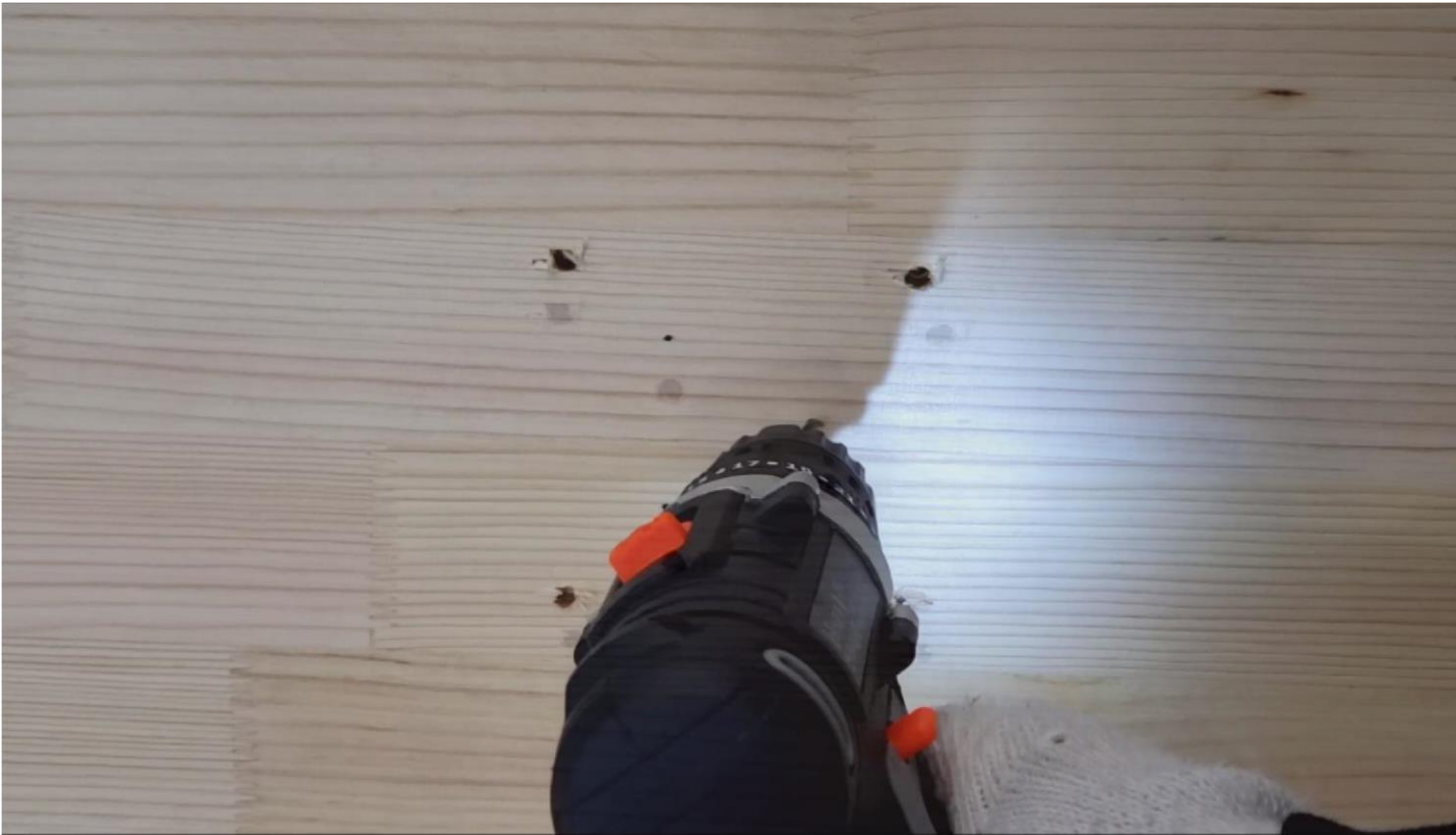
d) Drive in the expansion screw to the screw hole
