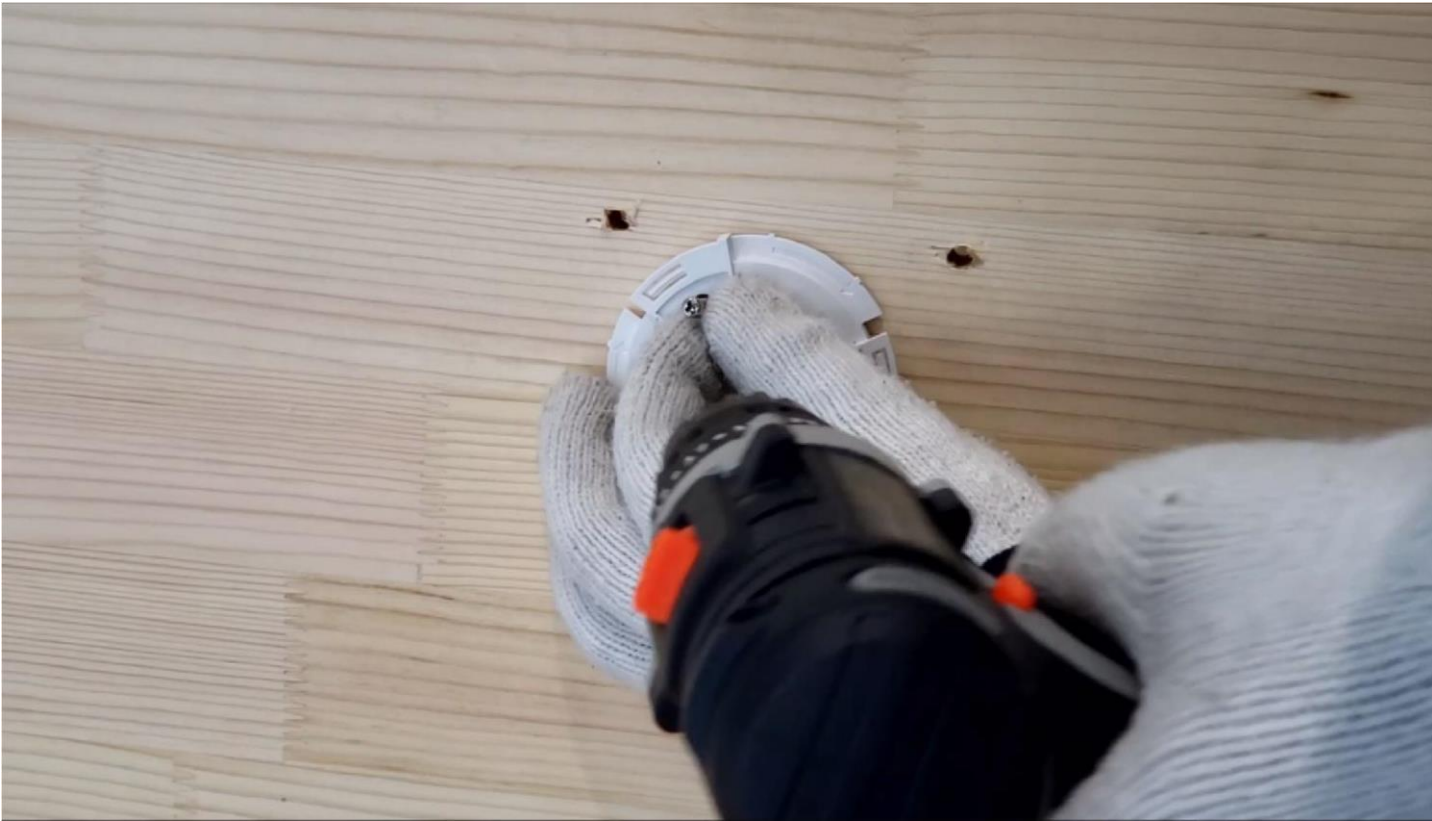
f) Remove side outlet and route the cable
