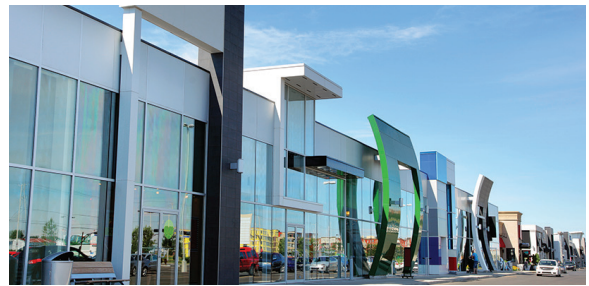
ENTRANCES TO COMMERCIAL BUILDINGS
